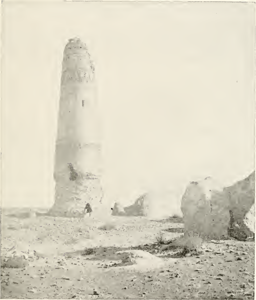
FIG. 118.—A Ruined Tower in Eastern Persia.
