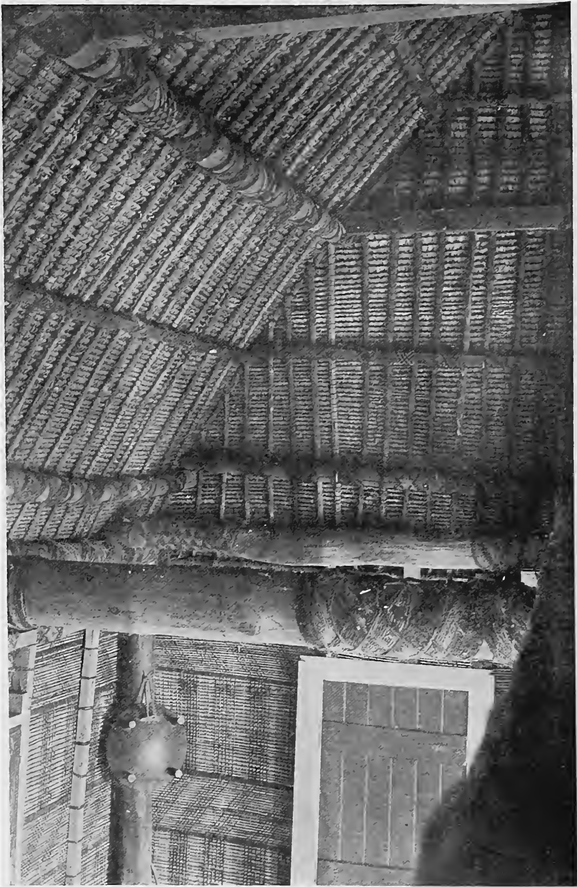
INTERIOR OF FIJIAN HOUSE, SHOWING HOW IT IS BOUND TOGETHER WITH COCO FIBRE
