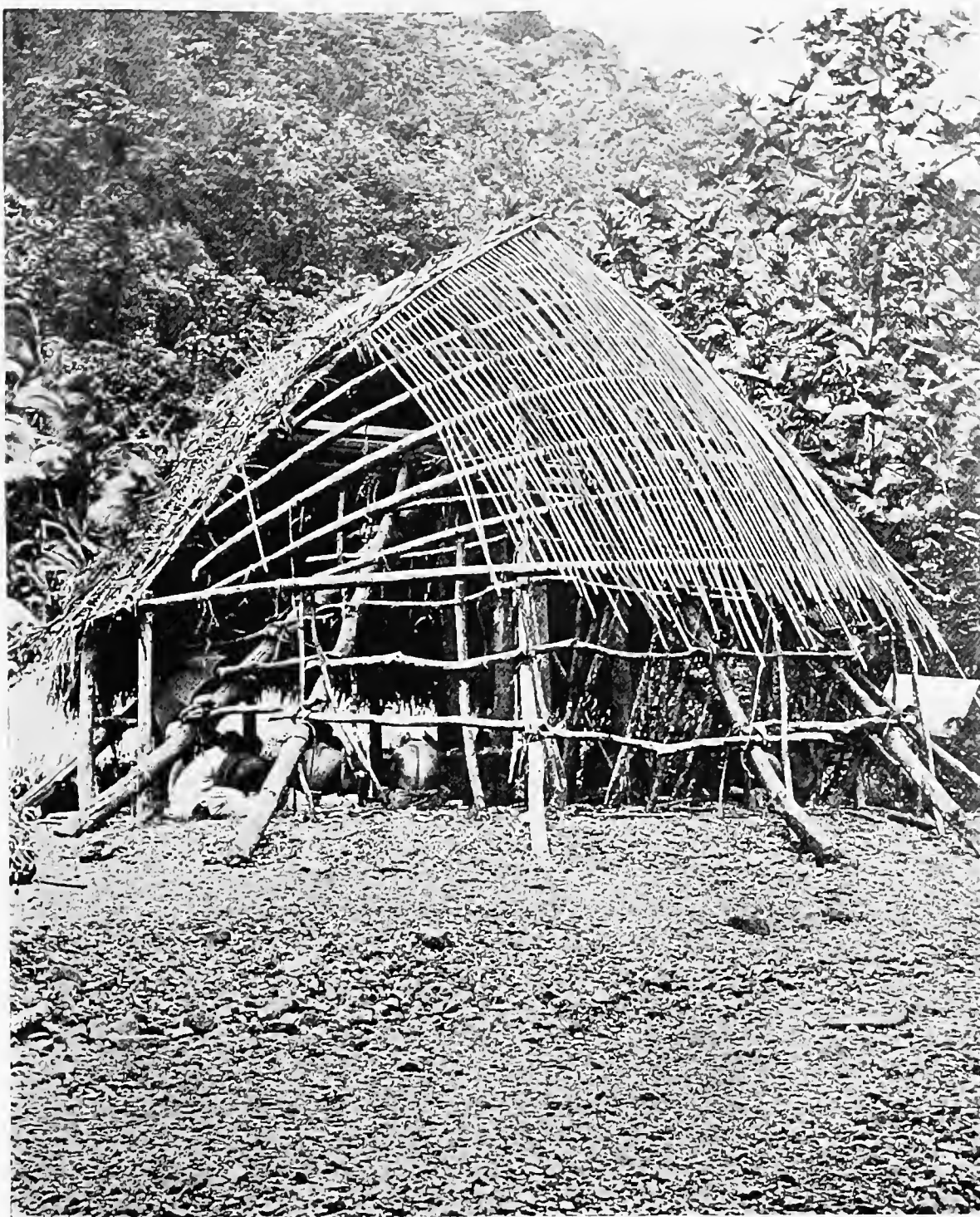
A SAMOAN HOUSE IN THE COURSE OF CONSTRUCTION
