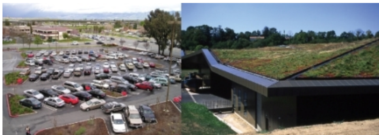
Figure 18.30: Impervious surfaces (left) fragment habitats, increase runoff, degrade water sources, reduce photosynthesis, and effectively increase CO 2 in the atmosphere. In the U.S., they cover an area of land almost the size of Ohio. Permeable pavements and green roofs (right) are beginning to reverse their effects. (14)
