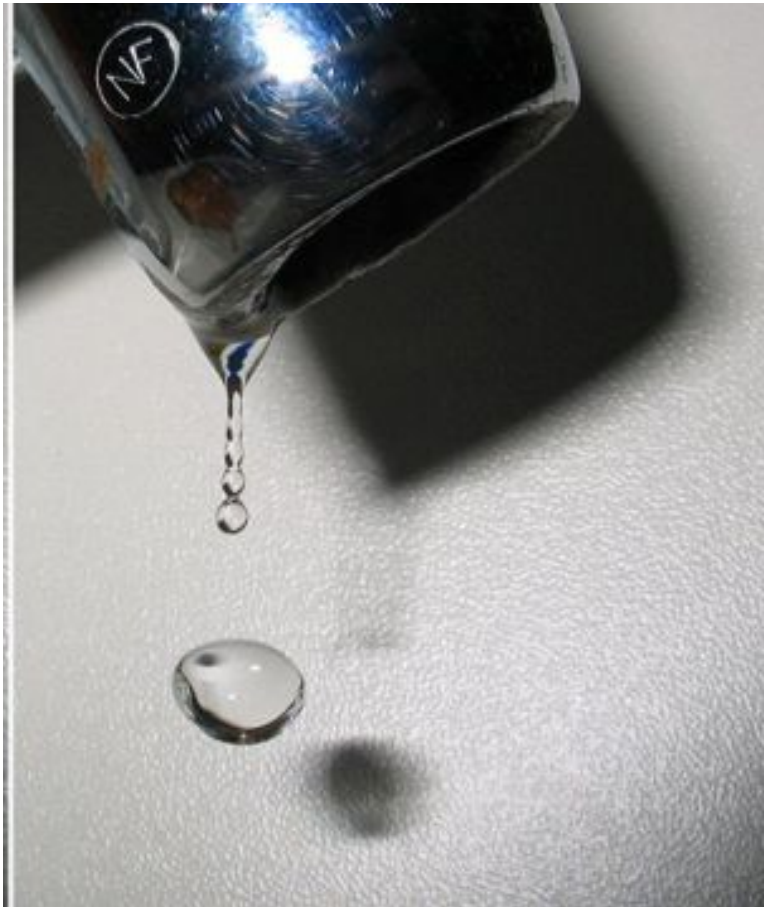
Figure 18.18: One drop per second from a dripping faucet wastes 2,700 gallons of water per year and adds to sewer and/or septic costs, as well. (27)
