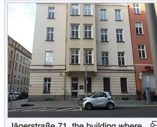
Jägerstraße 71, the building where José Rizal completed Noli Me Tángere , was the first building the Philippine government considered for the Embassy's permanent chancery
